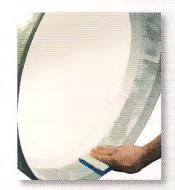
The dampened sponge will reactivate the adhesive to ensure zero air permeability.
